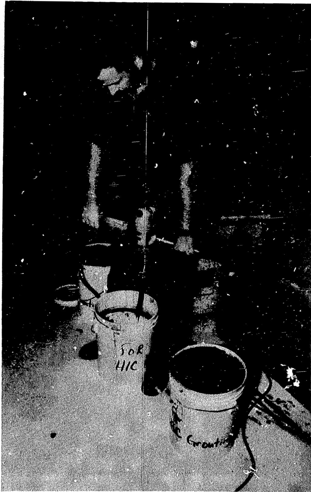
Figure 18. Photograph of epoxy concrete AEX-1512 grout being mixed outside hot shop.
