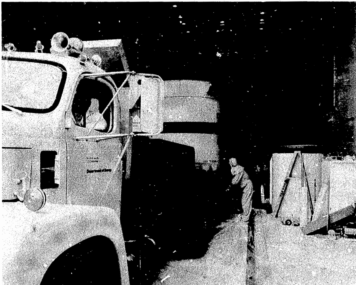
Figure 20. Photograph of trailer being disconnected from tractor in hot shop.
